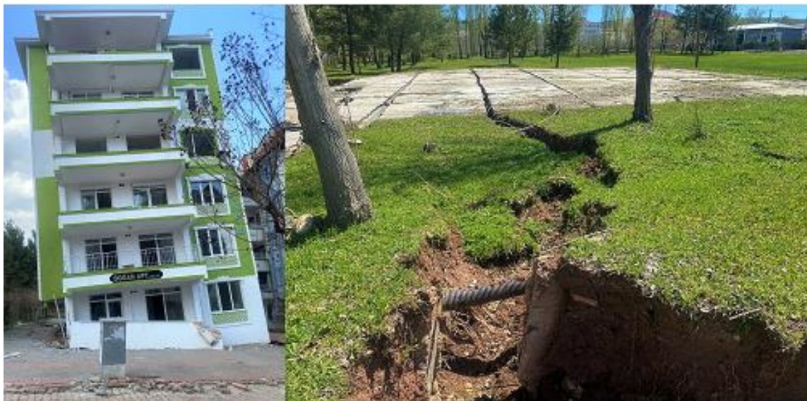
Slika 7. Primer utekočinjenja tal in delno nagnjena stanovanjska hiša v Gölbaşıju (levo). Površinski pretrg po potresu v Gölbaşıju, provinca Adiyaman (desno). (vir: 2023 Turkey–Syria earthquake - Wikipedia) Figure 7. An example of soil liquefaction and a partially tilted apartment building in Gölbaşı (left). Cracked land after the earthquake in Gölbaşı, Adiyaman Province (right). (Source: 2023 Turkey–Syria earthquake - Wikipedia)
