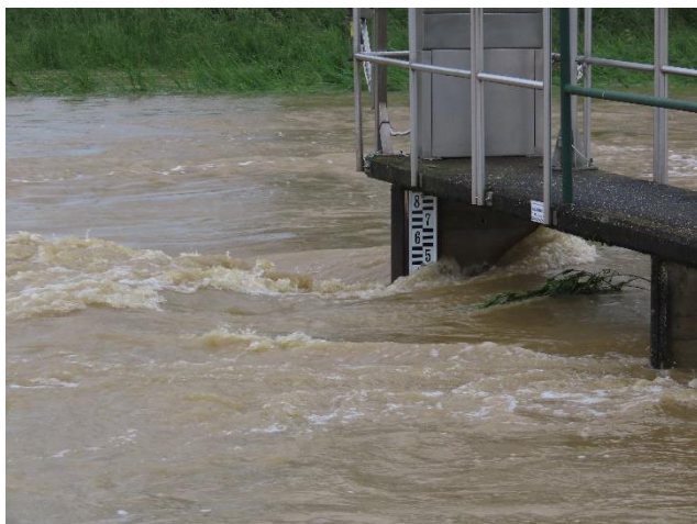
Slika 6. Pesnica v Zamušanih ob visokovodnem dogodku 17. maja 2023 z oznako najvišje izmerjene gladine vode v zgodovini meritev. Figure 6. Pesnica River in Zamušani during the high water event on May 17, 2023 with the mark of the highest water level in the history of measurements.
