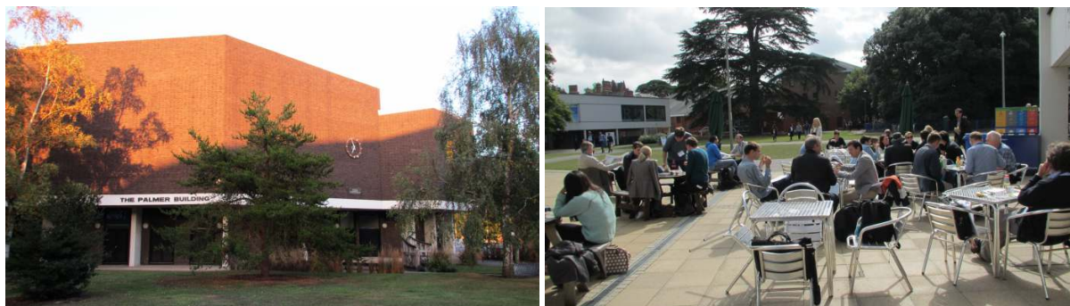
Slika 2. Konferenčni center in udeleženci pred stavbo v času kosila Figure 2. The Palmer Building and participants during lunchtime in front of the building
