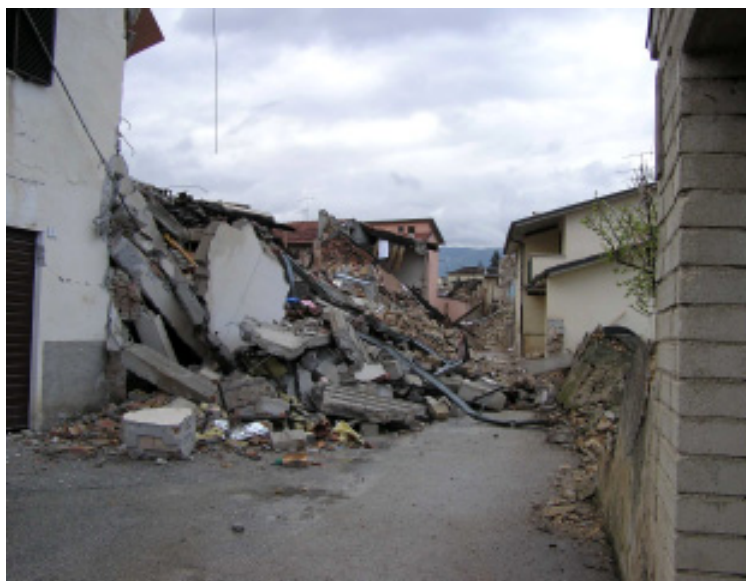
Slika 6. Ena izmed ulic v popolnoma porušeni vasi Onna (foto: I. Cecić) Figure 6. One of the streets in completely damaged village Onna (Photo: I. Cecić)
