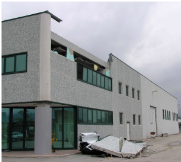
Slika 7. V novem delu vasi Monticchio je prišlo do poškodb na novih industrijskih objektih (foto: I. Cecić) Figure 7. Damage on the new industrial buildings in the the new part of the village Monticchio (Photo: I. Cecić)
